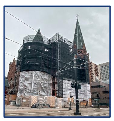
Most of the Phase 1 work was completed in late 2020 and was focused on the west side (front) of the building. The work included restoration of the stone facade, restoration of the four stained glass windows in the front doors, and restoration of four non stained-glass windows. The large stained-glass window over the front doors is part of Phase 1 and will be restored in early 2021 along with some cosmetic work on the steps and handrails. The bell tower is not part of Phase 1.
